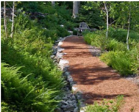
Infiltration trench parallelling a pathway.
