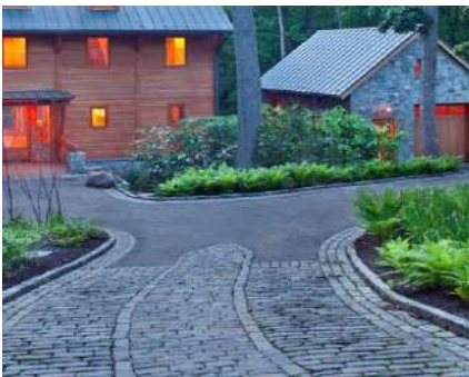
Banding asphalt driveway with stone.
