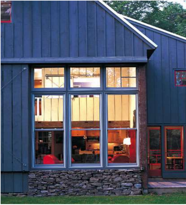
Fiber cement board siding with vertical battens.
