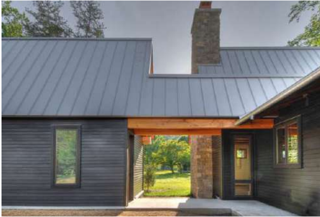
Wood siding oriented horizontally.
