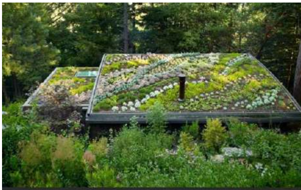
Vegetated roof slows stormwater runoff.
