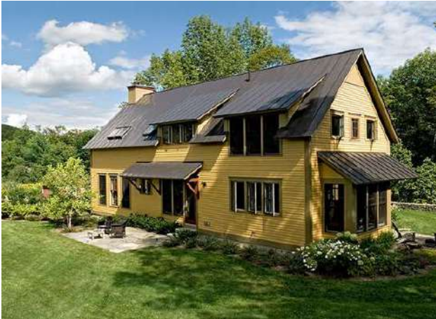
Standing seam metal roof with low sheen.
