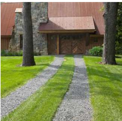
Tire track driveway reduce impervious service.
