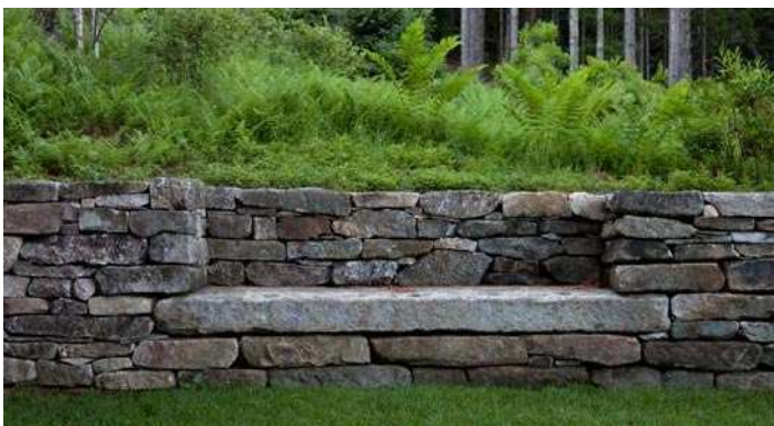
Simple bench constructed of indigenous stone.
