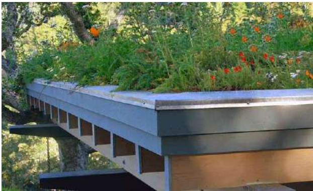
Vegetated roof limits solar heat gain and reduces runoff.
