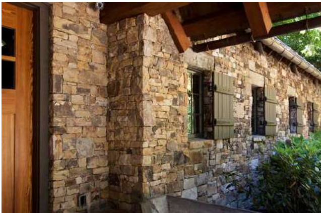
Indigenous dry stack stone exterior.
